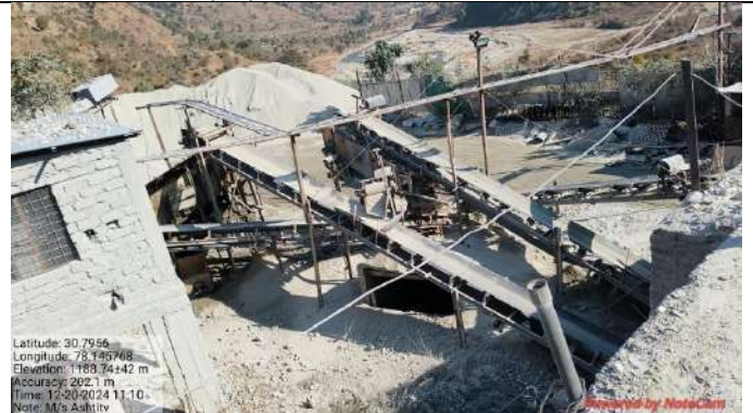
Pic. (04) Non-operational Stone Crusher
